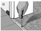
Leave an expansion space of approx. 5 mm between the board and the base of the moulding. As a rule, a fine saw must be used to cut a gap the thickness of a board in wooden door frames to allow the laminate floor to expand. Be sure to remove all distance spacers once all boards are laid. Fasten skirtings (with or without clip system) to the walls – that's it.
